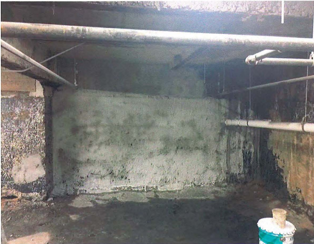
Basement waterproofing in progress
