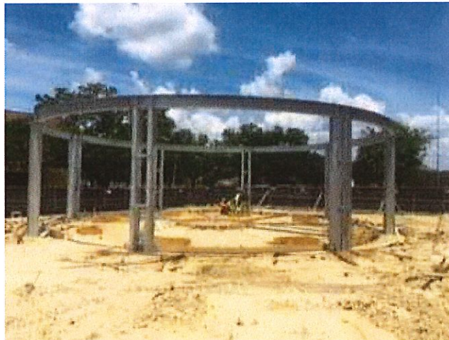
Construction in progress
