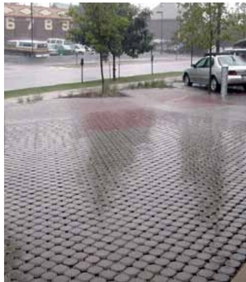
Permeable paving
