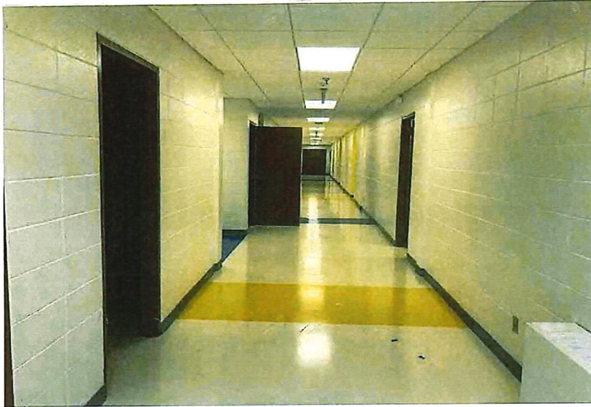
SUBR - Stewart Hall Renovations progress / proj. manager Kestee Weir III
