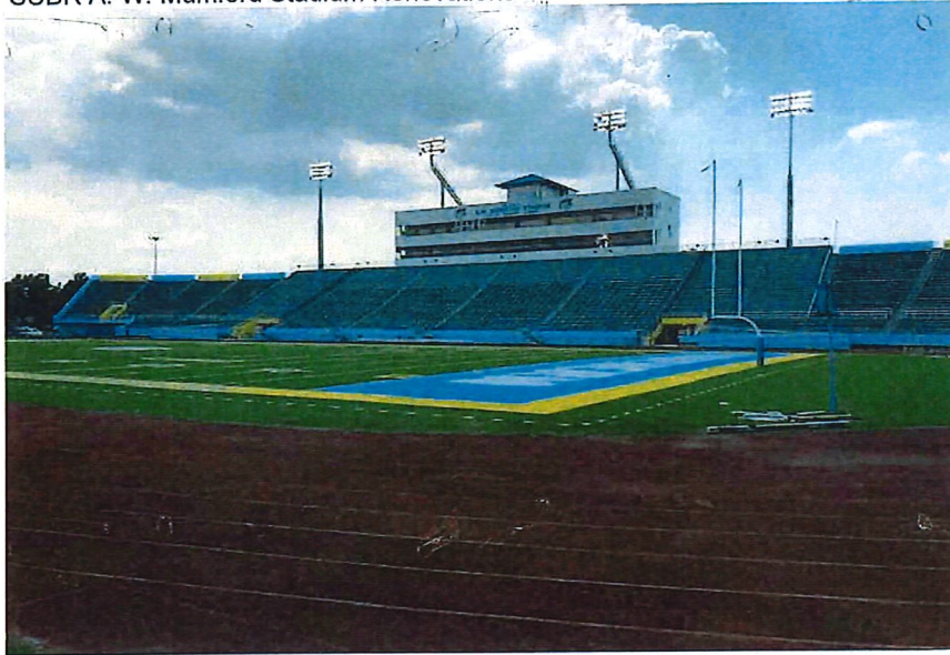
SUBR A. W. Mumford Stadium Renovations
