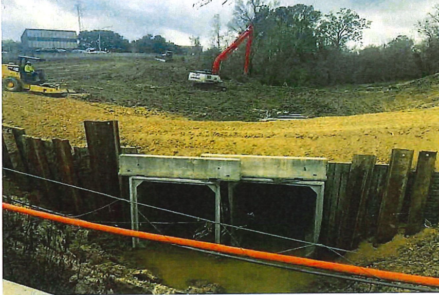
SUBR - Ravine Erosion Control System and Road Improvements in progress Dec. 2019
